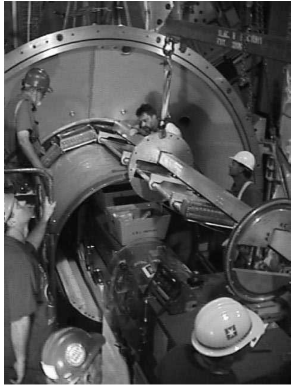
Figure 30. Installation of a bar box into the BABAR detector. Not seen in the figure is the cantilevered support arm which supports the installation fixture above the accelerator components.
