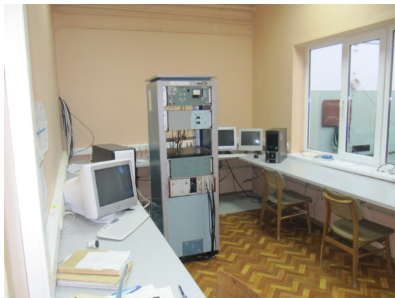
Figure 8: NESTOR facility control room.
