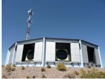
Figure 6: FD building at Los Leones during the day. Behind the building is a communication tower. This photo was taken during daytime when shutters were opened because of maintenance.
