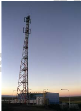
Figure 12: One of the five communications towers: the one shown is deployed at the Los Leones site; see Figure 11.
